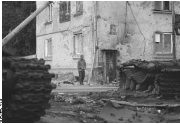
A man stands near a damaged building in South Ossetia's capital. With the Georgian assault crushed by Russian troops, ethnic Georgian villages have paid the price.
