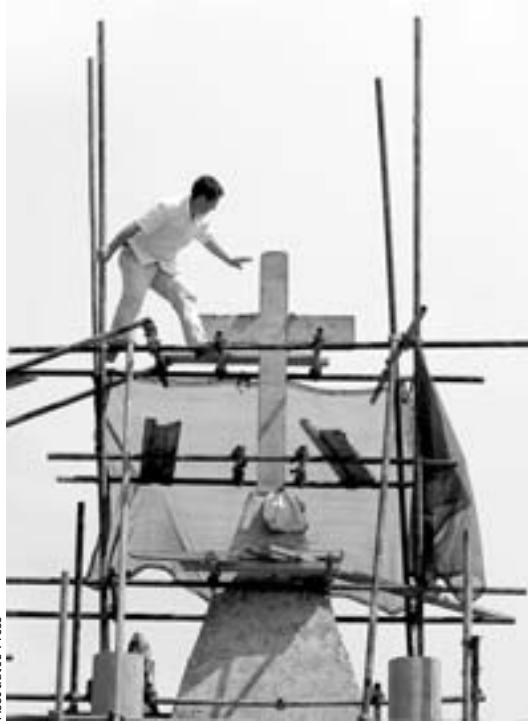
A church under construction in Huaian in east China's Jiangsu province.
