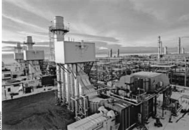
Technology at Exxon Mobil's La Barge, Wyo., facility strips carbon dioxide from natural-gas wells and reinjects the greenhouse gas underground.
