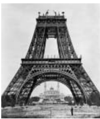
The Eiffel Tower during its construction in the late 1880s.
