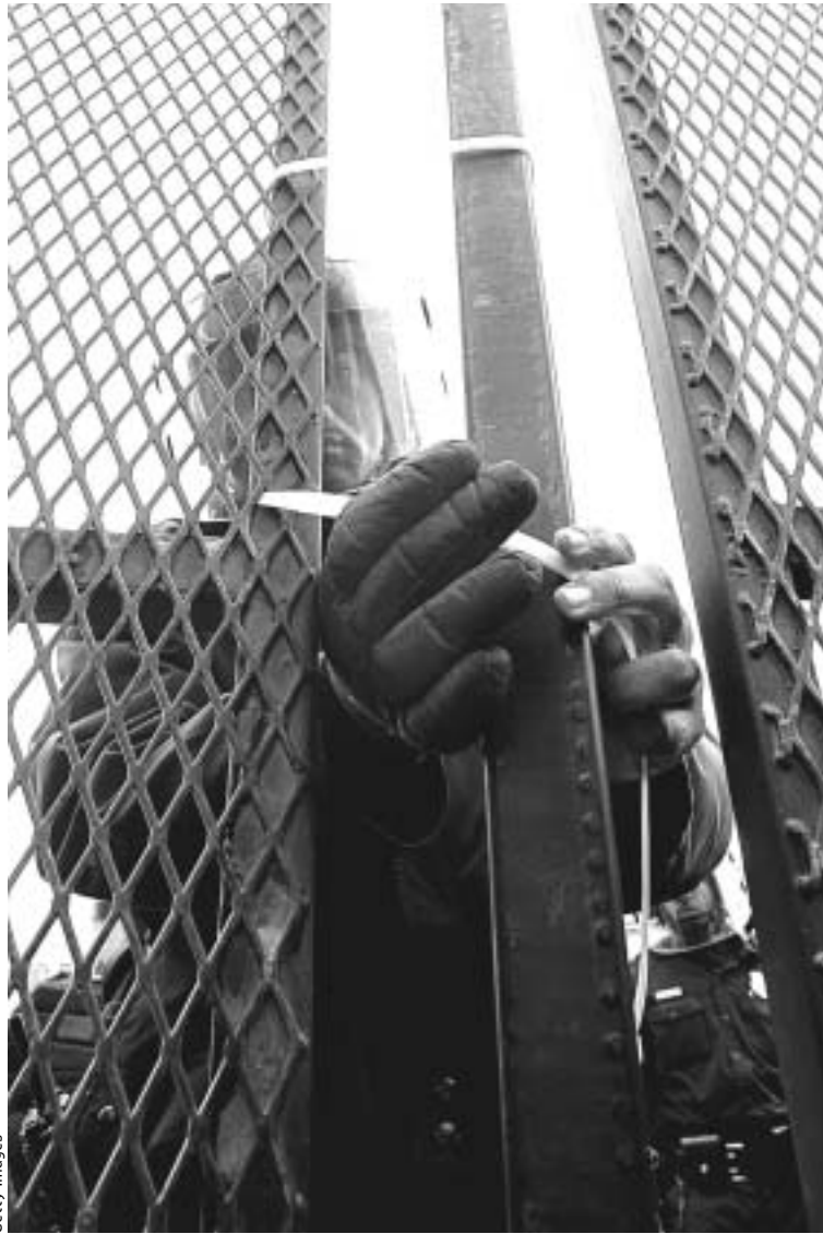
During the 2005 U.S. inauguration, a tip that fences weren't secure wasn't passed onto police. Protesters easily toppled the fences , which were then mended.
