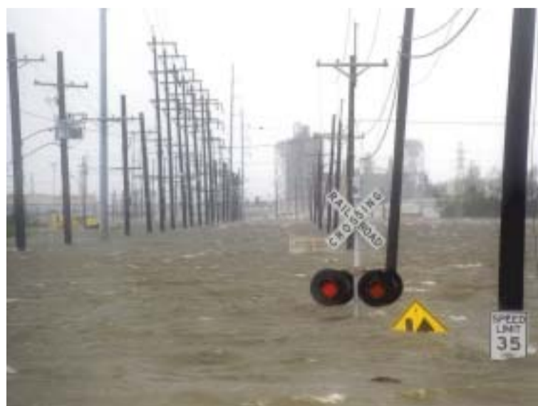
A railroad crossing is inundated by floodwater caused by Hurricane Gustav that surged over the side of a levee on the Industrial Canal in New Orleans.
