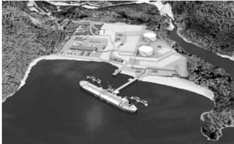
The Kitimat liquefied-natural-gas export terminal in British Columbia, shown in a rendering, is expected to be completed by early 2014.
