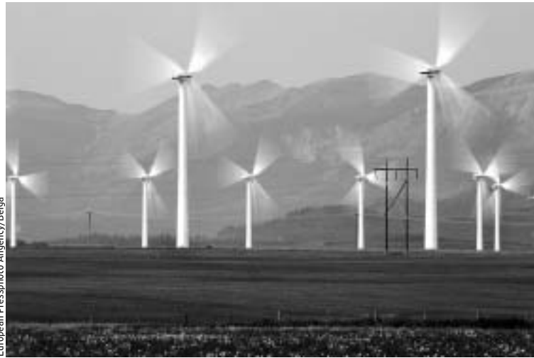
Vestas wind turbines turn in the wind at Cowley Ridge Windplant in Alberta, Canada
