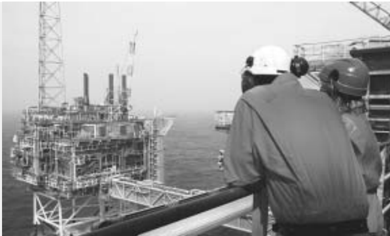
Workers at StatoilHydro platform Sleipner T, in the North Sea off the coast of Norway
