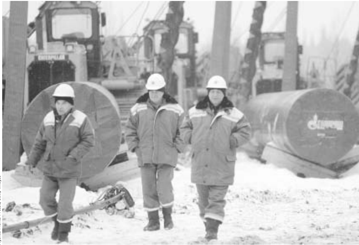
Pipeline workers at Gazprom's Bovanenkovo project, the largest gas field in the Yamal Peninsula of Siberia, in December.
