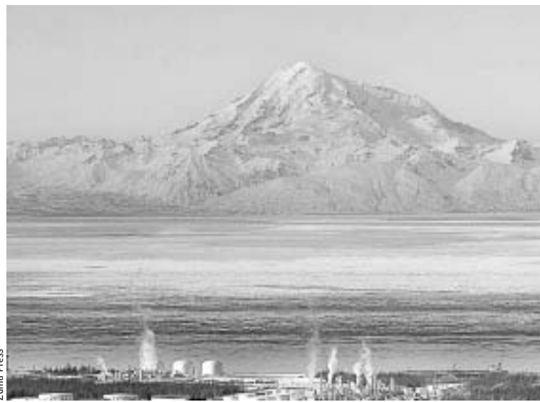
Conoco's LNG facility in Alaska sits in the shadow of Mount Redoubt.
