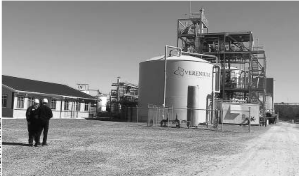
BP and Verenum's new Louisiana demonstration refinery, above, produces ethanol from sugar-cane stalks. Their planned Florida facility will be 25 times larger and produce the biofuel from grasses.
