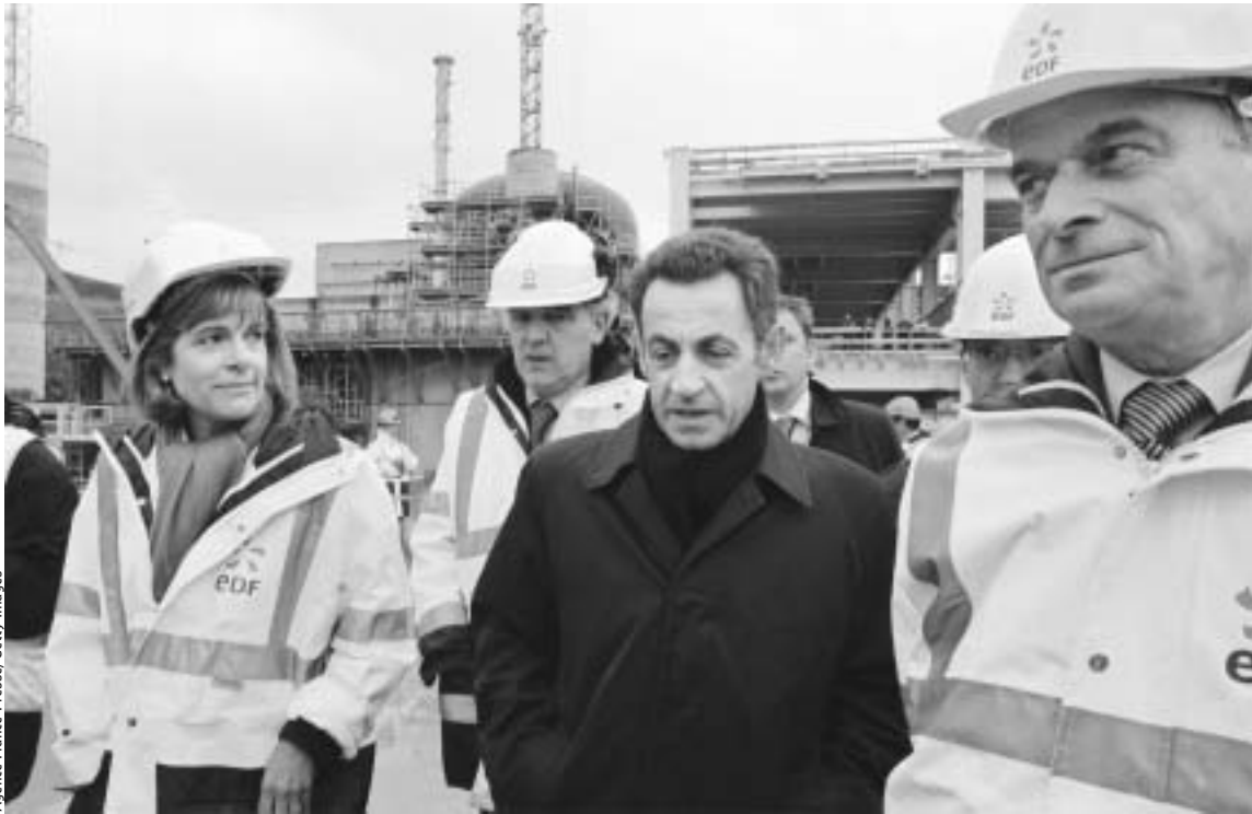
Areva CEO Anne Lauvergeon and French President Nicolas Sarkozy, center, tour a French nuclear plant under construction.
