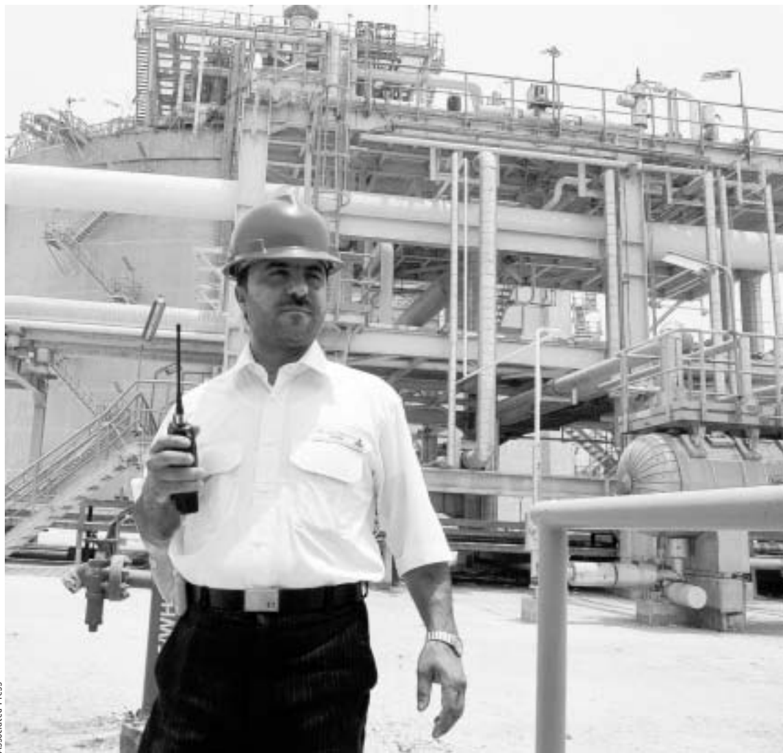
A worker walking on the grounds of a partially built facility at Iran's giant South Pars gas field in July. Officials have said they will suspend activity at the Pars LNG project.
