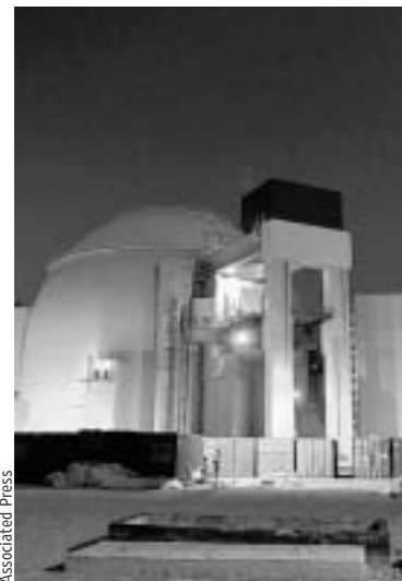
Iran's Bushehr nuclear power plant.
