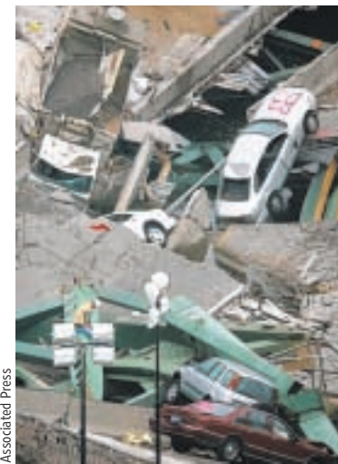
A Minneapolis bridge collapsed in '07.
