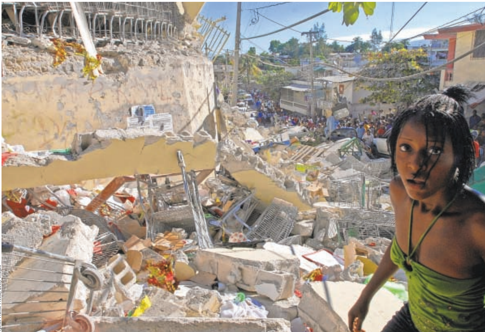
Buildings in Port-au-Prince were reduced to rubble. The port itself collapsed, making it hard for large shipping vessels to dock.
