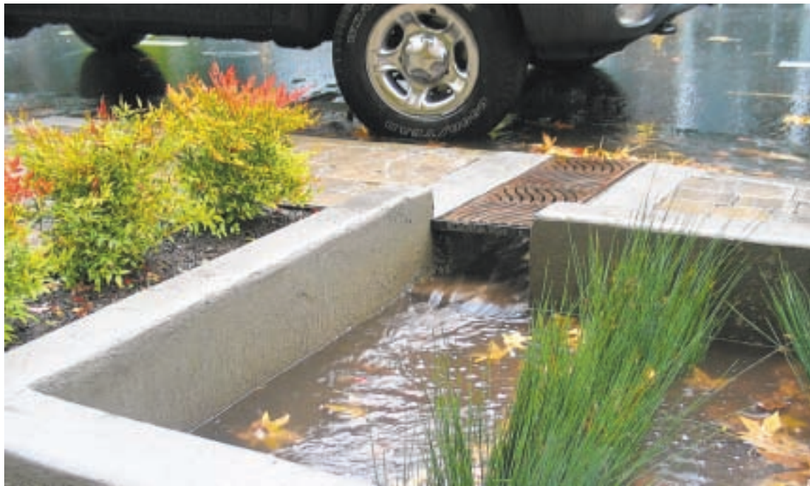
Rainwater flows into a sidewalk planter from a street in Portland, Ore.
