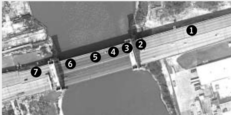
Note: Locations are approximate, based on Michael Hunter's testimony Source: Justice Department; Bridge image: Google Earth
