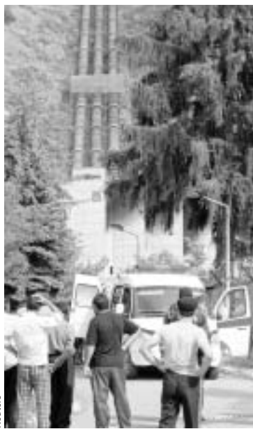
The station's damaged turbine hall.
