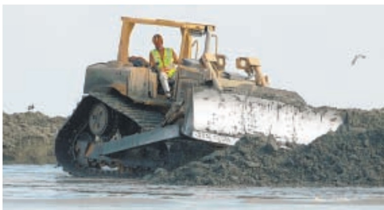
A bulldozer builds up a barrier on East Grand Terre Island, La., this week.
