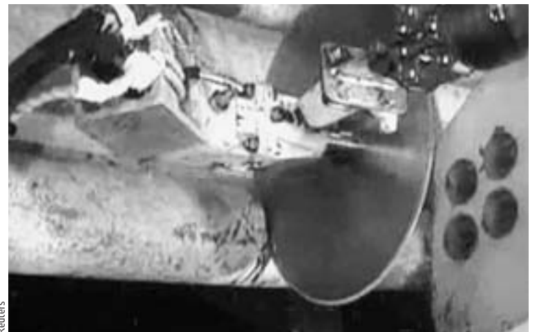
Technicians use a robotic saw at the site of the Deepwater Horizon oil leak.
