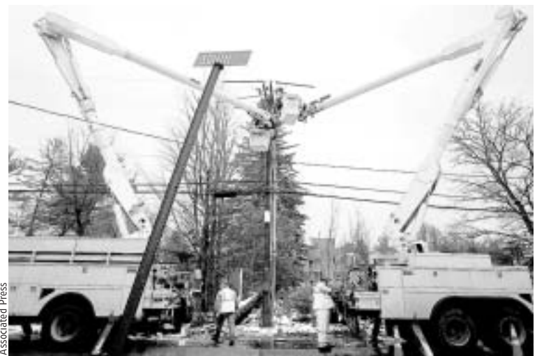
Crews work to restore electricity last month in Bow, N.H.
