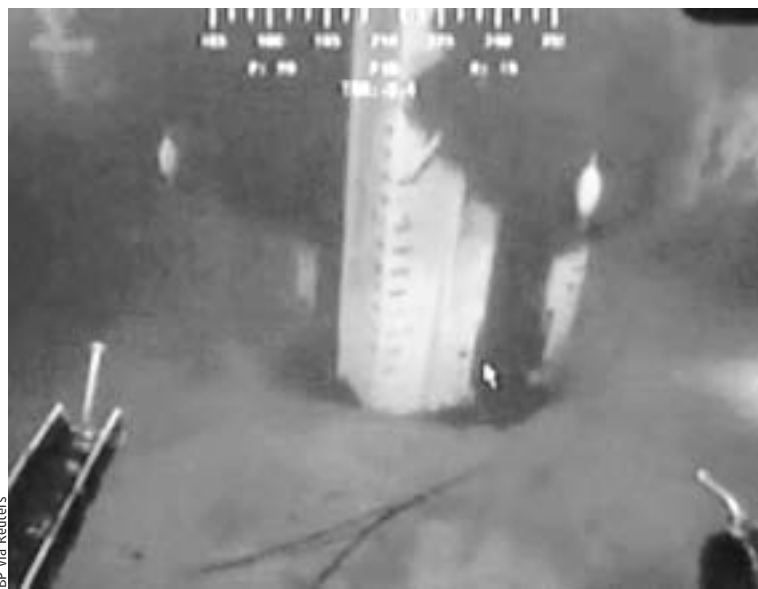
A containment dome is placed over a leak at the seafloor. The effort failed.
