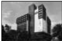
Park Lane by CMP Taichung, Taiwan
