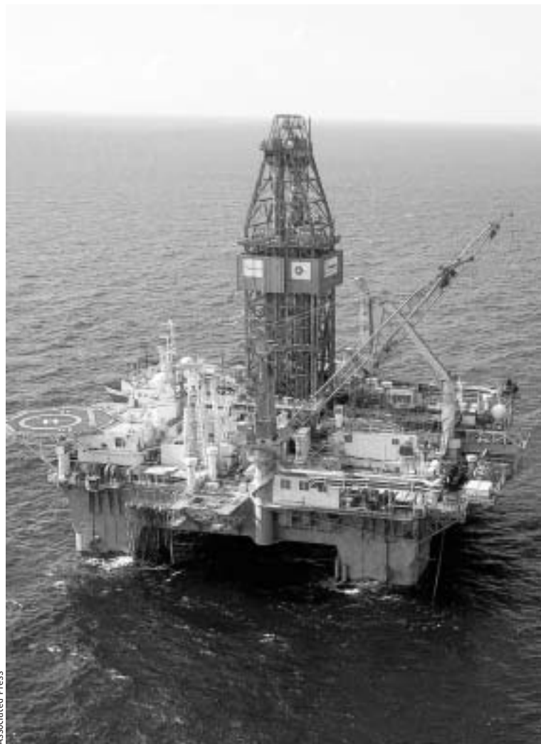
A driller worked on the relief well to seal BP's oil spill in the Gulf of Mexico.
